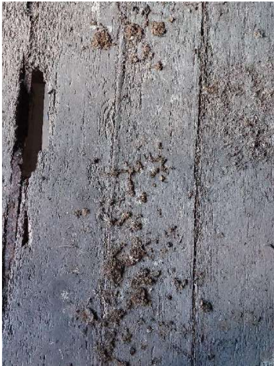
Fig 3.80: Heavy decay to timber floorboards
