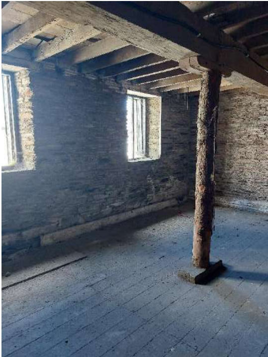
Fig 3.56: View of south east corner.
