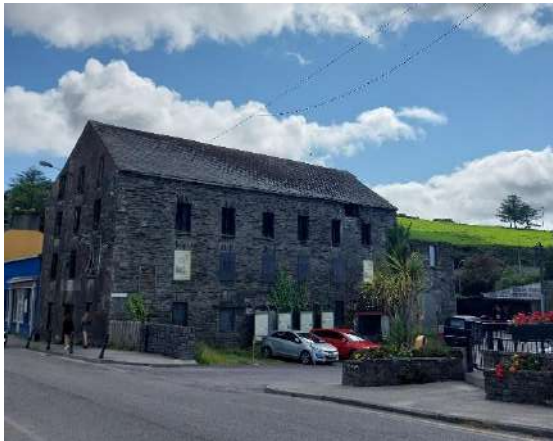
Fig 3.02: View of mill from Ilen street
