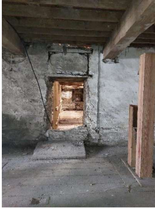
Fig 3.60: Door opening into south annex with failed lintel above.
