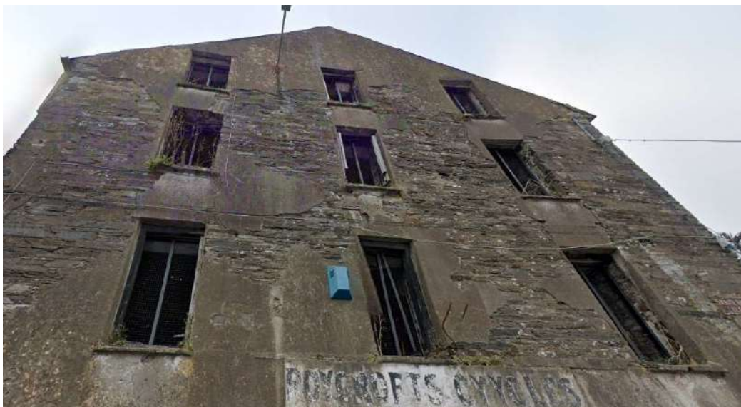
Photo 7 – Eastern gable out of plumb
