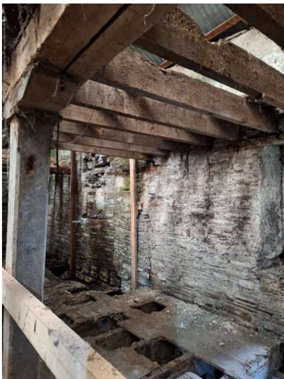
Photo 19 – West facing wall requiring replacement
