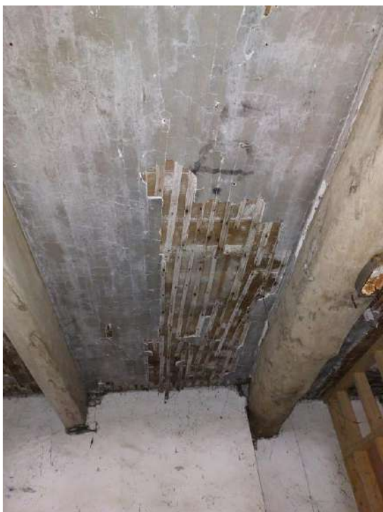
Fig 3.64: View of ceiling in west room with lath and plaster visible.
