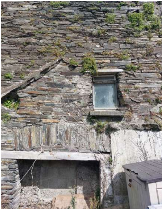
Fig 3.21: View of west elevation with former roof line, former opening and modern window opening.
