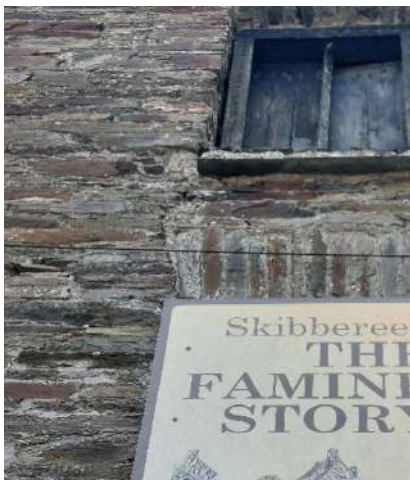
Fig 3.12: Cracking above window
