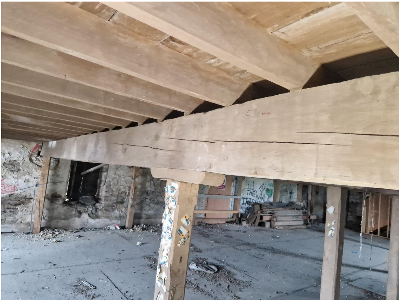
Figure 9. Shows a typical girder. Note the shake in the timber along the grain. This has little weakening of the timber section.
