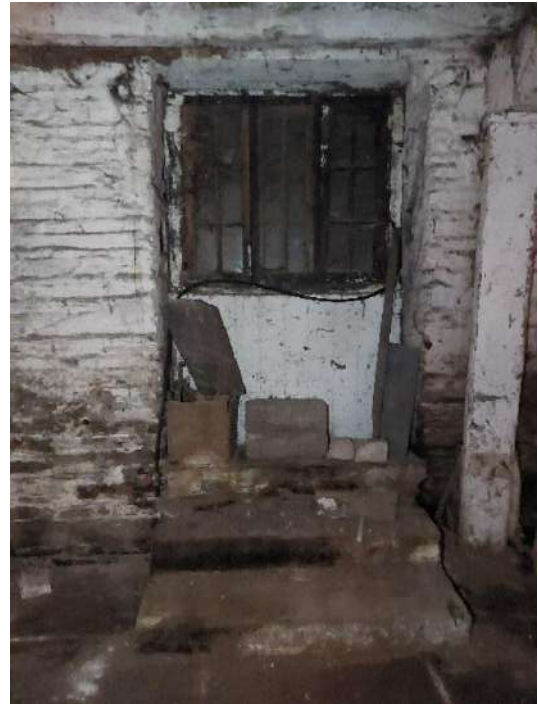
Fig 3.96: Door opening in south gable wall of annex
