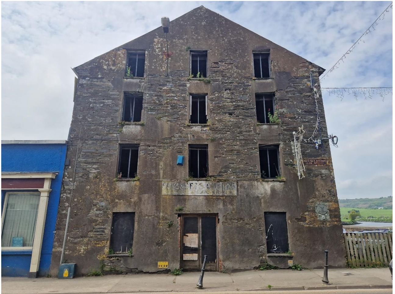
Figure 4. Shows the main gable fronted elevation of the building. Note that as there are no windows present, water penetrates and decays the lintels. Most lintels on this elevation have decay present.
