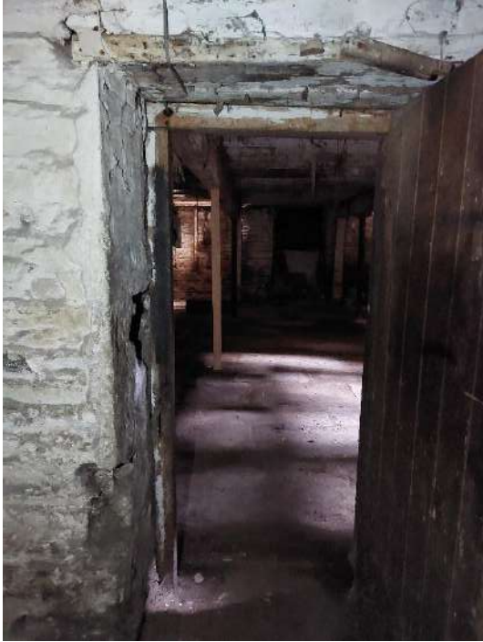
Fig 3.41: Door into south annex
