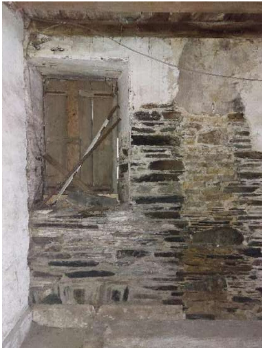
Fig 3.62: View of north wall of main room adjacent to masonry partition wall. Timber shutters to window. Differing section of stonework visible.
