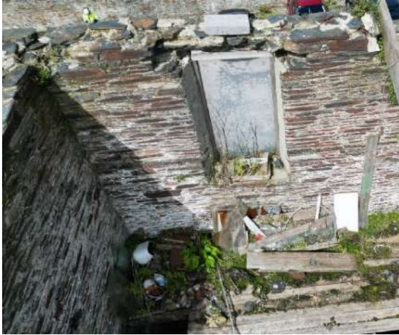
Fig 3.19: Loose masonry to top of walls
