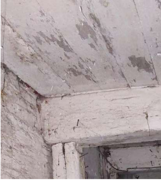
Fig 3.32: Timber beam embedded in damp external walls to south side of main volume.
