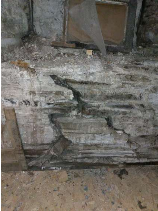
Fig 3.93. Cracking to south gable wall between openings
