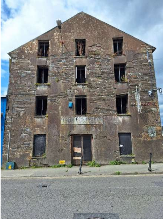
Photo 1 – Main mill warehouse east elevation
