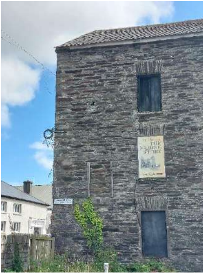
Fig 3.10: North east corner
