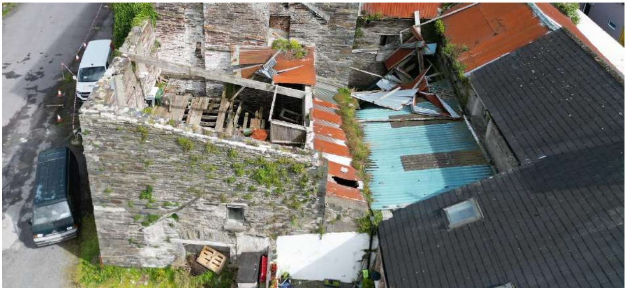
Fig 3.18: View of west annex
