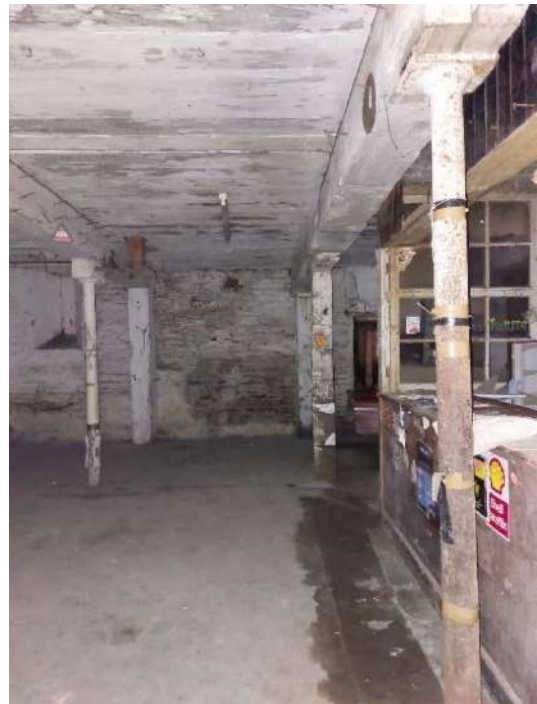
Fig 3.38: View towards south wall of main volume. Shop to rhs.
