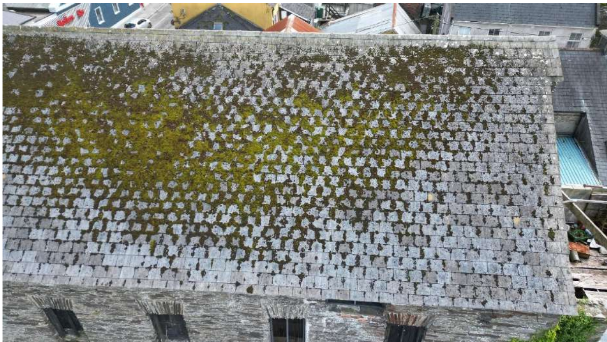
Fig 3.04: North face of roof of mill.
