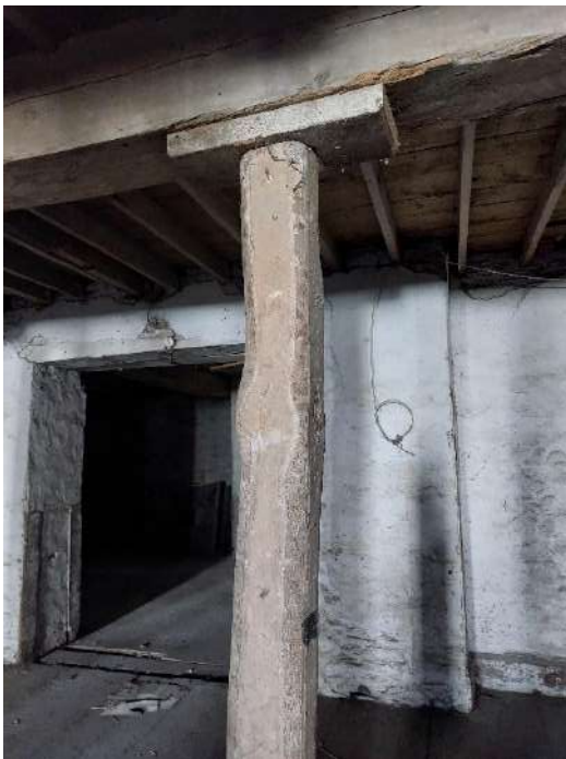
Fig 3.59: Column towards west formed by roughly hewn tree trunk with plate above visible.
