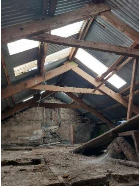
Fig 3.89: Roof structure of south annex
