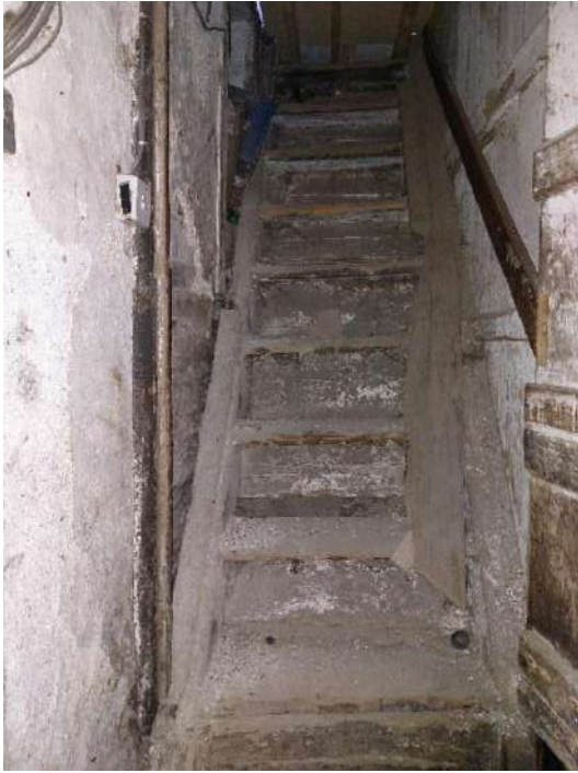
Fig 3.45: Historic timber stairs along north wall.
