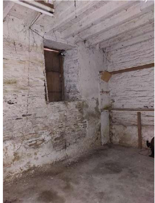
Fig 3.44: Window opening to east wall. Damp visible to lower section of wall.
