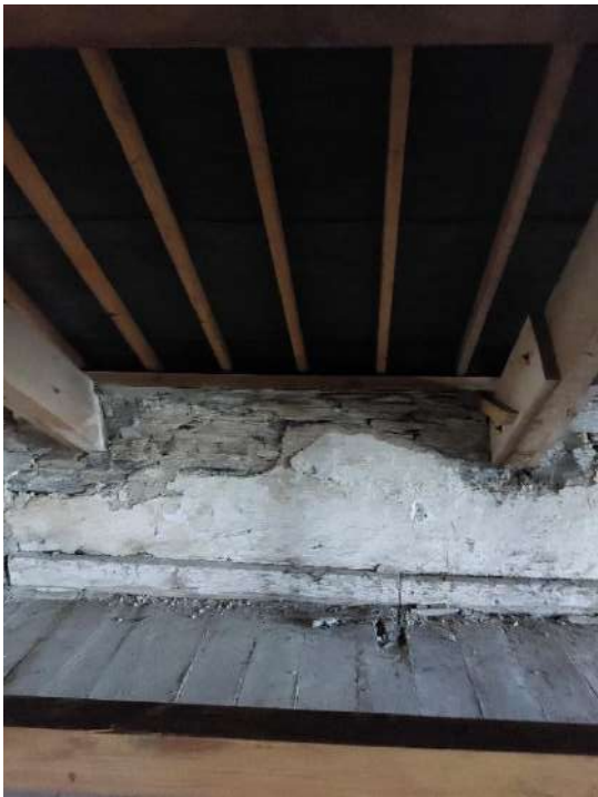
Fig 3.83: View of north wall
