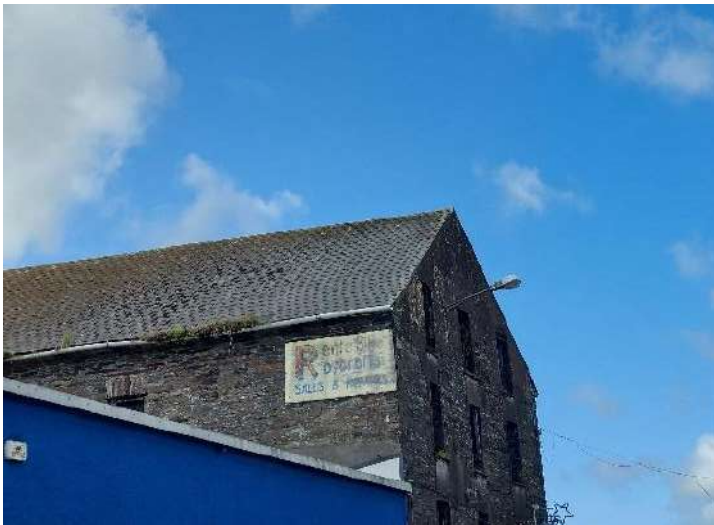
Fig 3.17: South elevation of main volume towards east corner.
