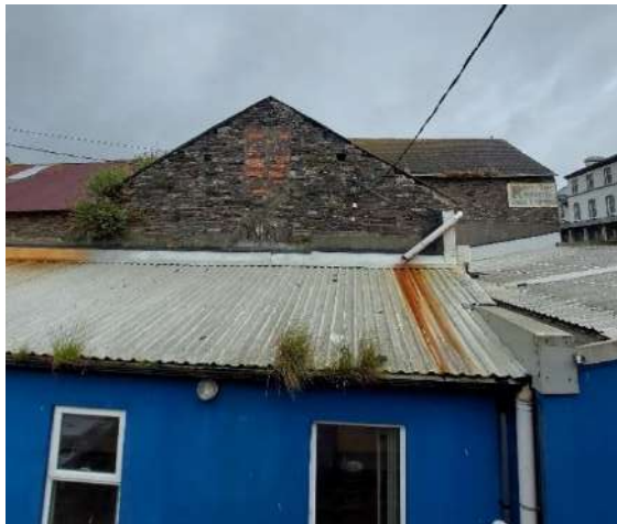
Fig 3.03: View from south of mill.
