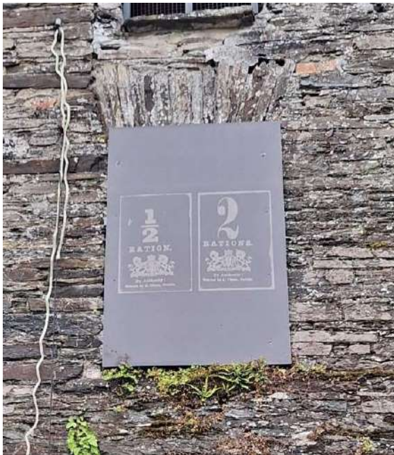
Photo 9 – Failed window head
