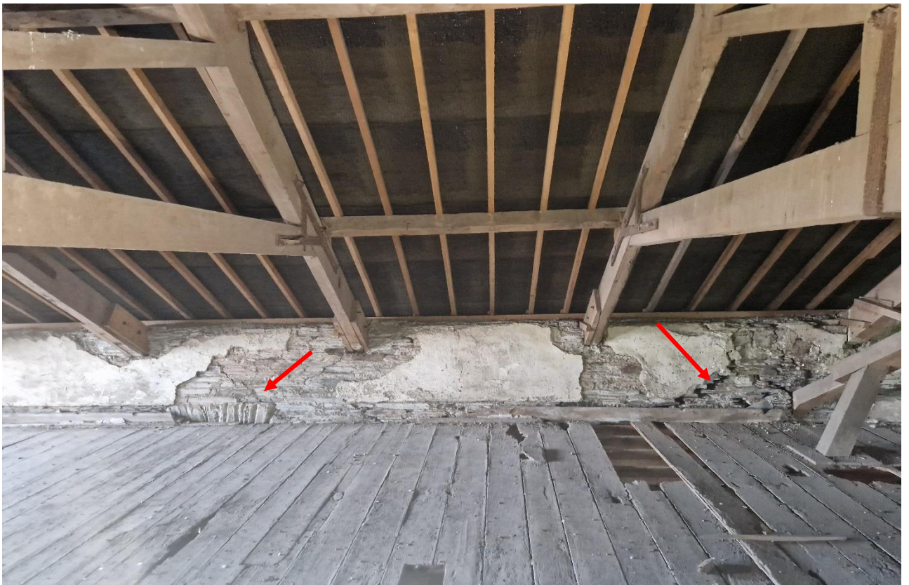
Figure 12. Shows a broad view of the roof detail. Note the masonry deflection where the lintel/arch failed.
