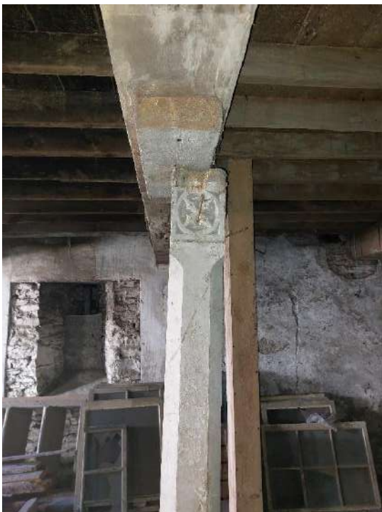
Fig 3.57: Misaligned column possibly from a church.
