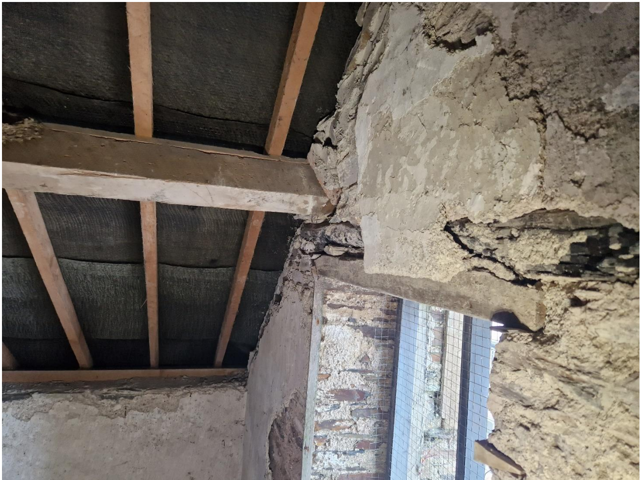
Figure 10. Shows displacement of the masonry around the purlin end.
