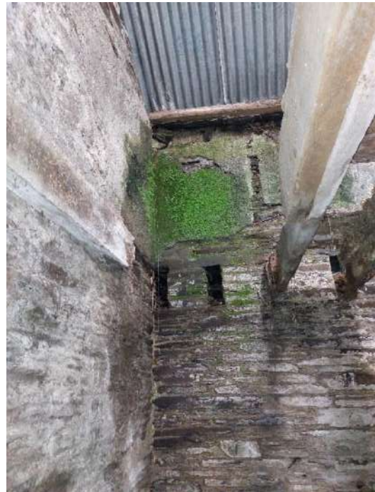
Fig 3.98 Mould and algae growth visible on west wall
