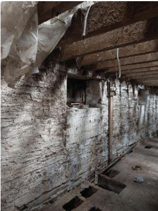
Fig 3.94: View of east wall
