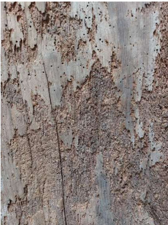
Fig 3.70 Detail of woodworm damage to beam
