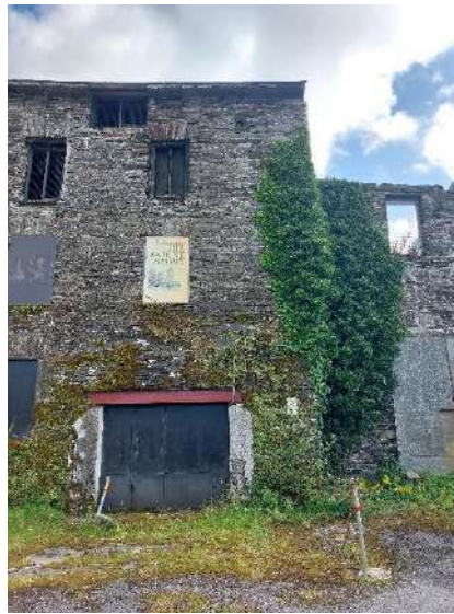
Fig 3.14: View of north west corner of building – significant ivy growth visible
