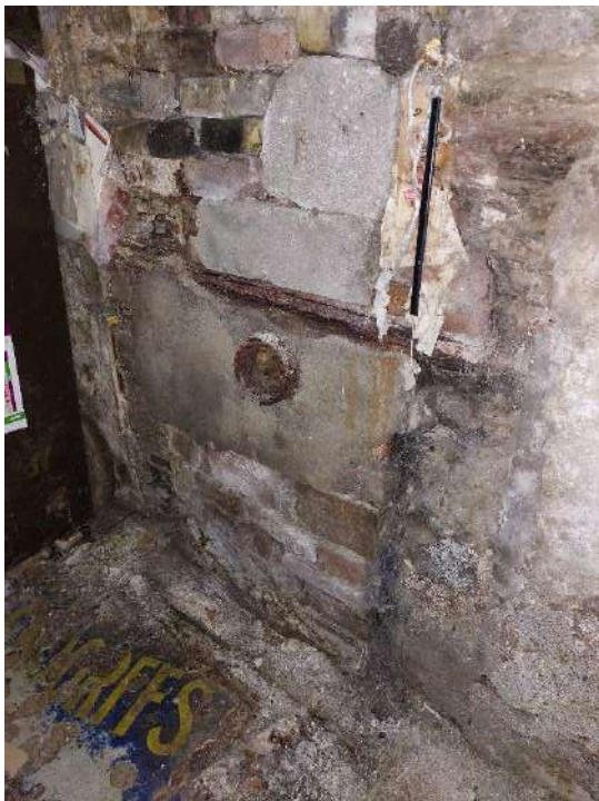
Fig 3.46: Possible former flue / chimney to north wall in shop area.
