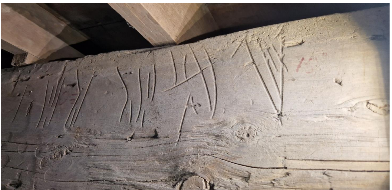
Figure 14. Shows typical baltic marks visible on some timbers.
