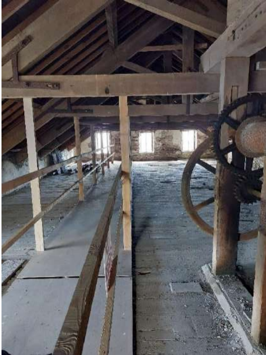
Fig 3.75: View of third floor facing east
