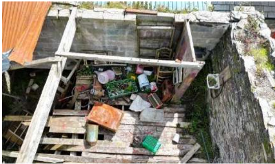
Fig 3.20: Concrete block wall to south elevation
