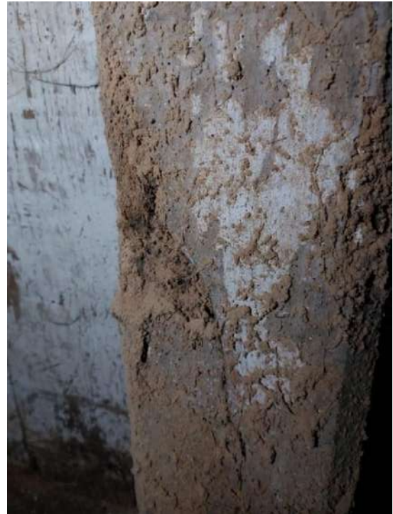
Fig 3.36: Significant woodworm infestation to timber column
