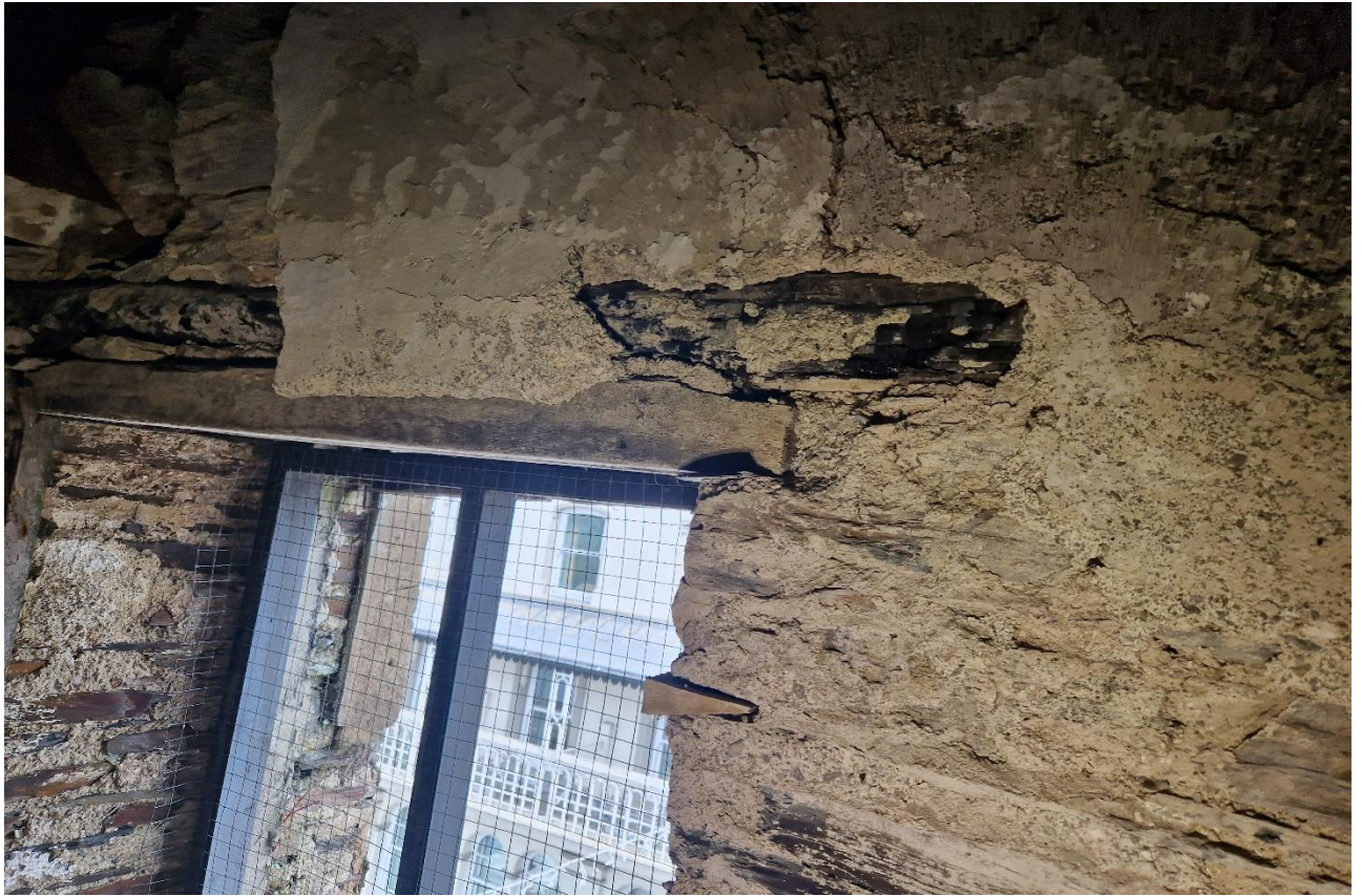
Figure 5. Shows a double lintel at the third-floor level. Note the upper lintel has fire damage.
