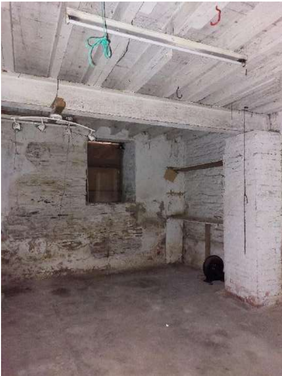
Fig 3.26: Northeast corner of ground floor. Modern floor structure above supported on brick piers. Damp visible to walls.
