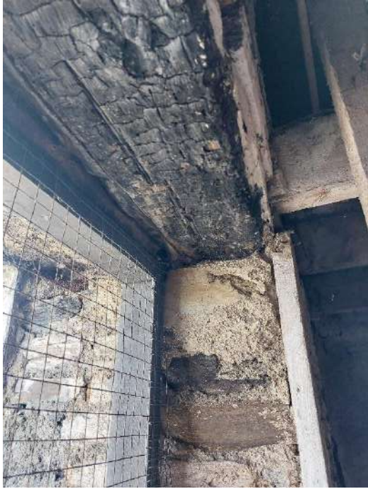
Fig 3.72: Charred timber lintel in east wall
