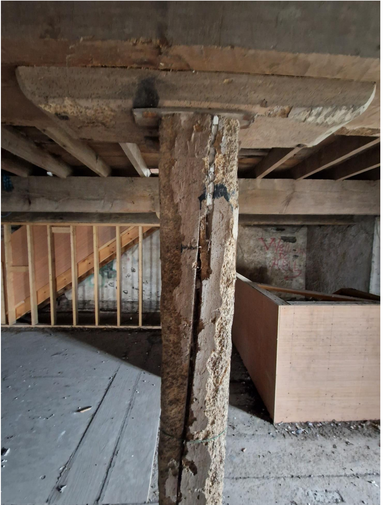
Figure 3. Shows heavy surface deterioration from active woodworm infestation. There is currently enough remaining timber for this post.
