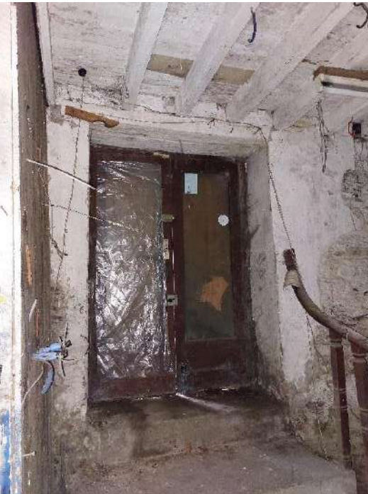
Fig 3.43: Door opening to east onto Ilan Street
