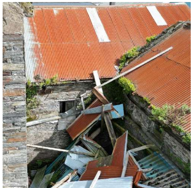
Fig 3.23: West wall of south annex with adjoining failed roof structure
