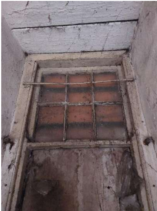
Fig 3.47: Sliding sash window to north elevation towards east of building.
