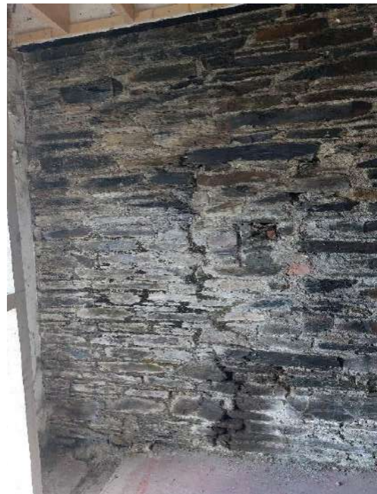
Fig 3.52: Some cracking visible to partition wall between main volume and west room.
