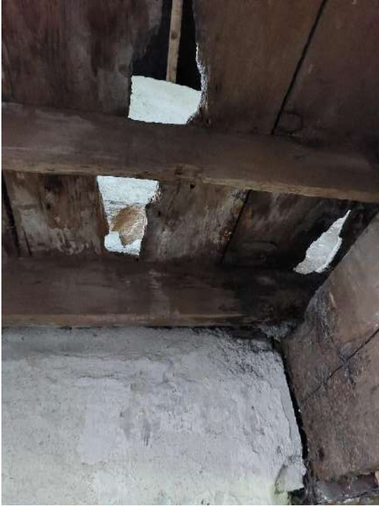
Fig 3.71: Boards forming ceiling very heavily decayed.
