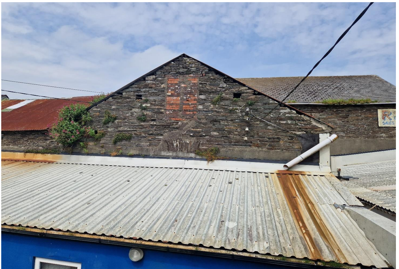
Figure 2. This highlights the poor condition of the south-facing gable.
