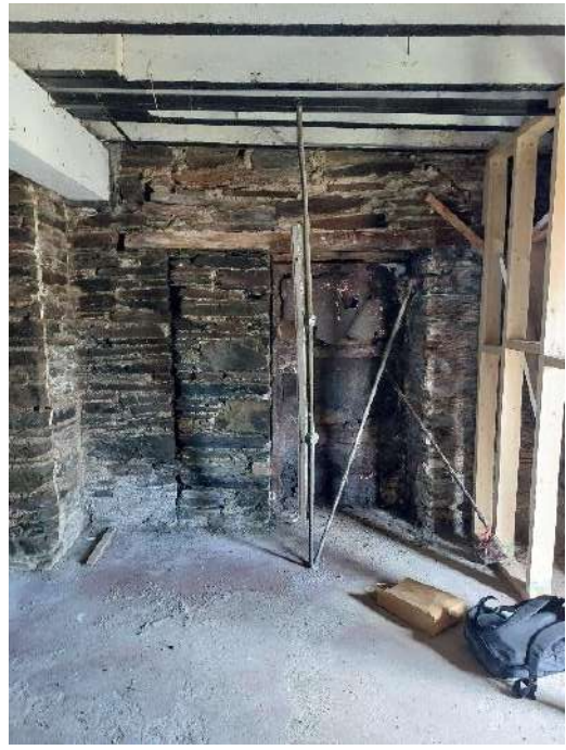
Fig 3.51: Former opening to west wall partially filled in in stone with decayed timber lintel above.
