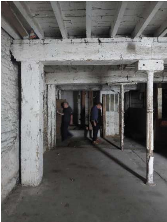
Fig 3.28: View towards west. Original timber structure visible.
