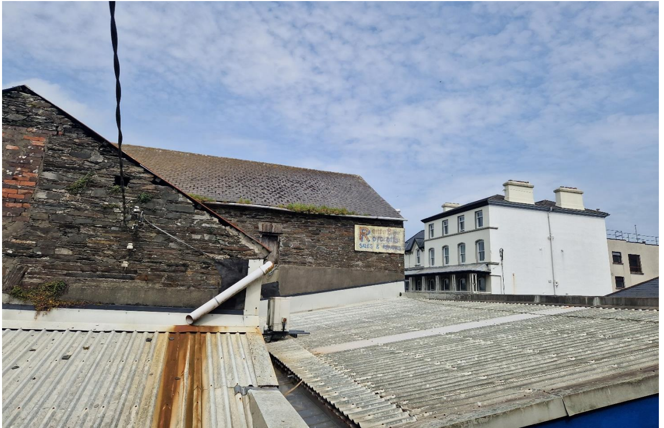
Figure 1. Highlights the heavy vegetation growing from the gutter, causing water to cascade down the face of the building.
