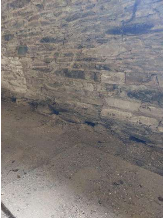
Fig 3.58: Top of former putlog holes visible to east wall at floor level.
