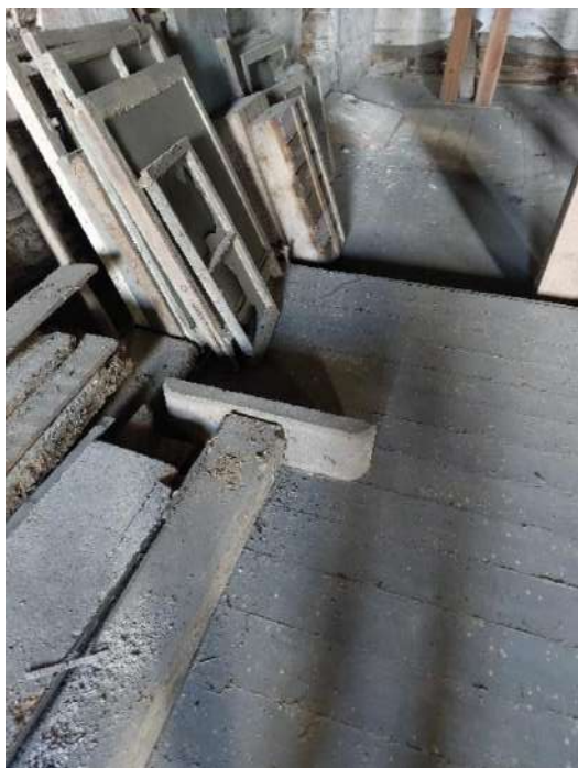
Fig 3.63: Fittings stored on first floor.
