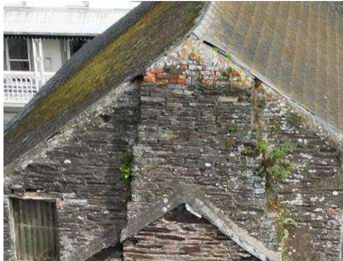
Fig 3.05: View of verge to west gable- note gaps visible between roof finish and walls.
