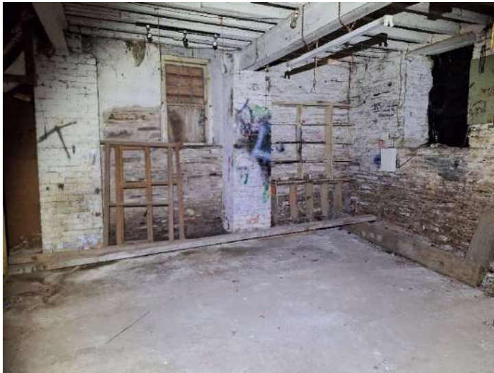
Photo 11 - Concrete ground floor showing steel beam and brick column supporting first floor
