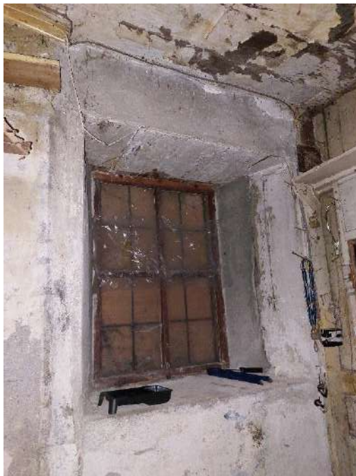
Fig 3.48: Timber window to shop area (west of building) with concrete construction visible around opening.
