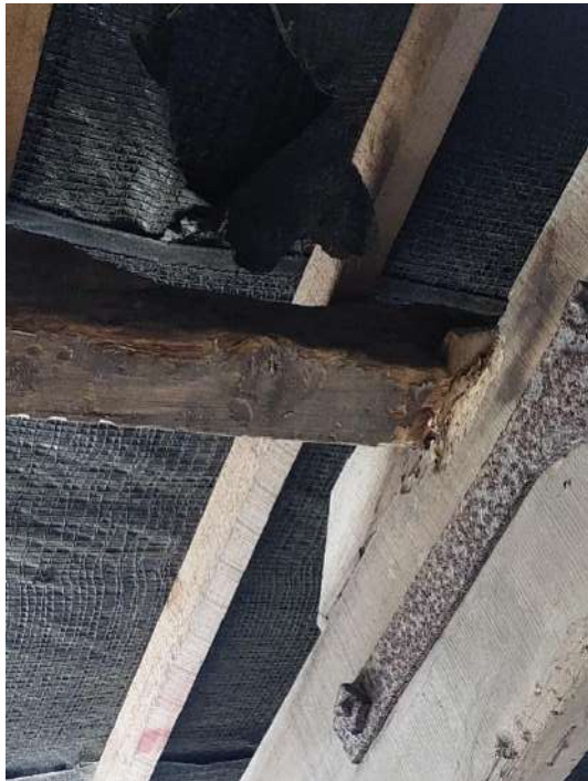
Fig 3.79: Decay visible to roof purlin
