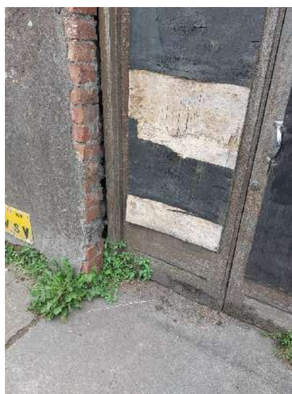
Fig 3.08: Door to east elevation
