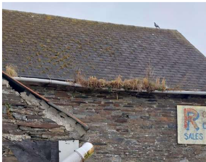
Fig 3.06: Gutters to south elevation. Significant vegetation and sagging visible.
