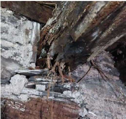
Fig 3.34: Decayed joist ends in west room
