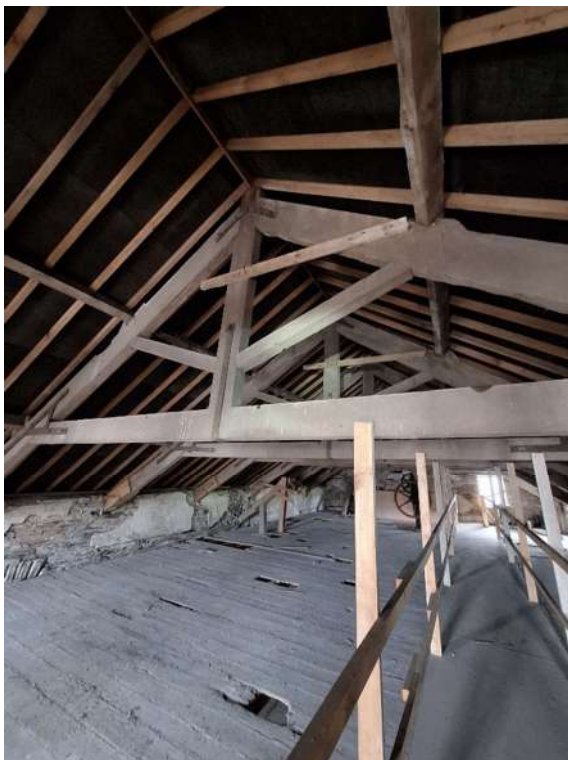
Photo 5 – Original roof truss
