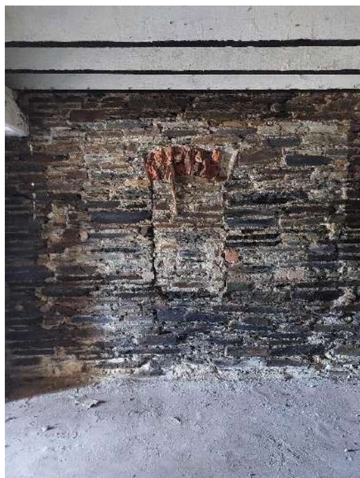
Fig 3.511: Former window opening into main volume now filled in. Brick arch above with significant spalling visible.
