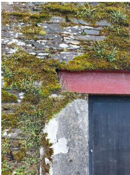
Fig 3.13 : modern steel lintel and significant moss growth
