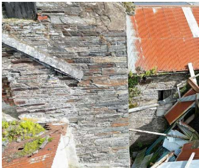
Fig 3.16: Southwest corner. Some render visible at eaves level. Lead flashing to former roofline visible.
