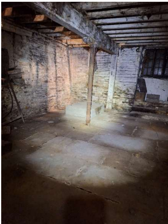
Photo 21 – Original paving slabs
