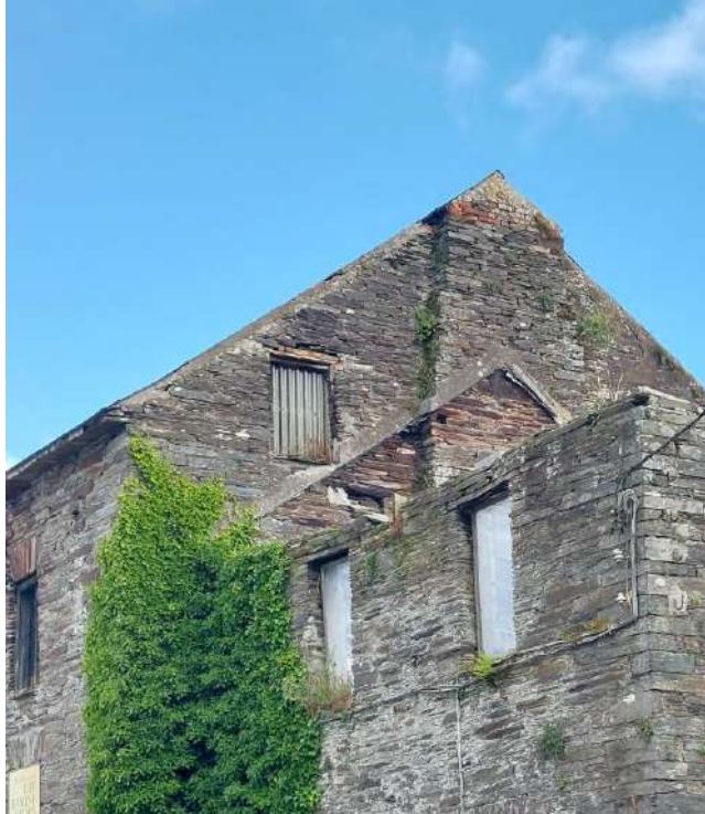
Fig 3.17: West elevation: eroded joints and cracking visible to north west corner, along with a significant amount of ivy growth.
