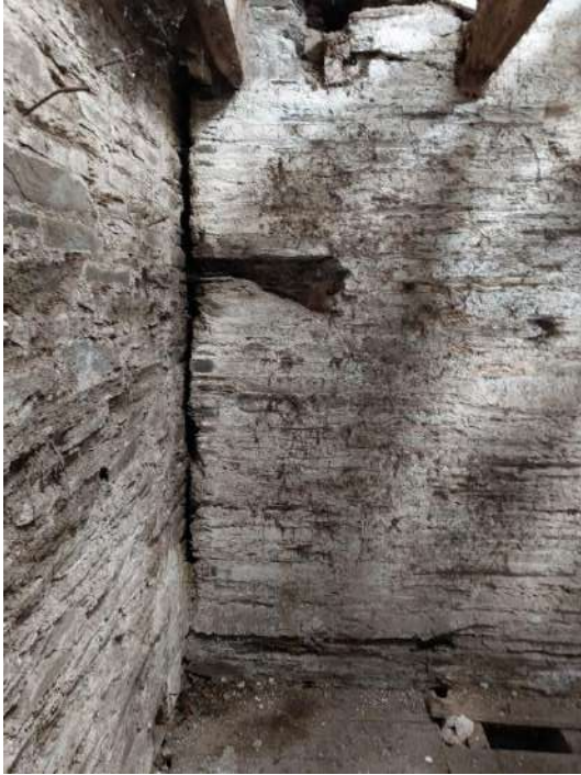
Fig 3.95: Crack at first floor level between main volume and south annex
