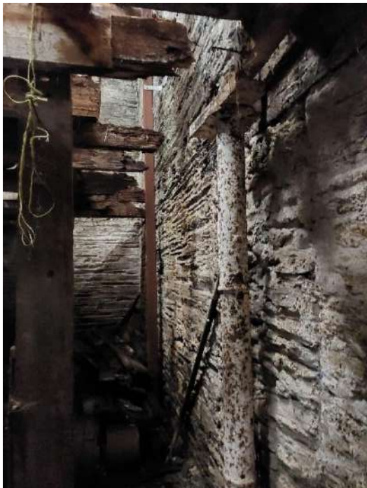
Fig 3.92. Decayed ends to floor joists along west wall
