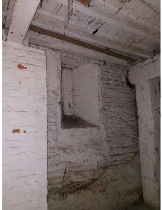
Fig 3.42: Closed up window opening to south wall.
