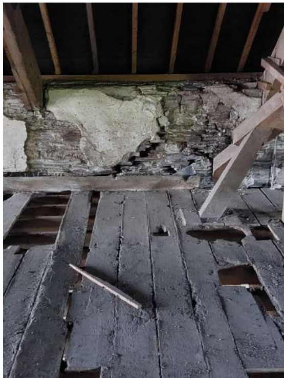
Fig 3.81: View of cracking to south wall which appears to be associated with the south annex.
