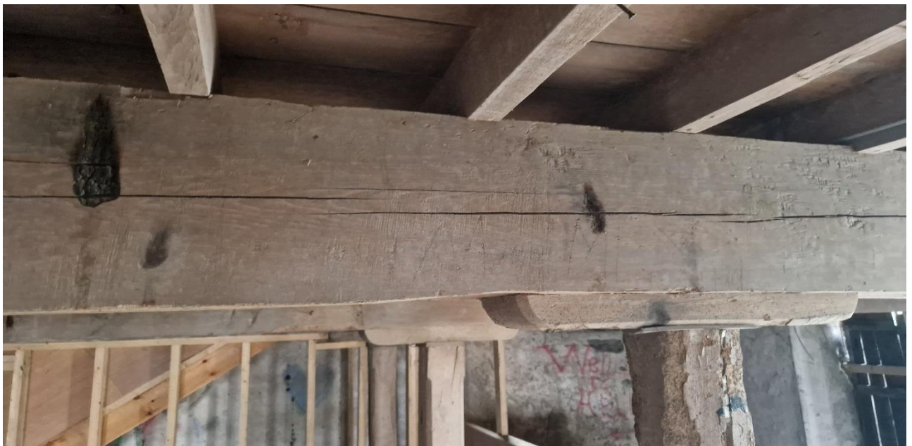
Figure 13. Shows two of several burn marks present in the building.
