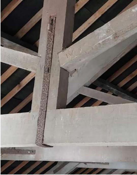
Fig 3.78: Timber truss with carpenter marks visible
