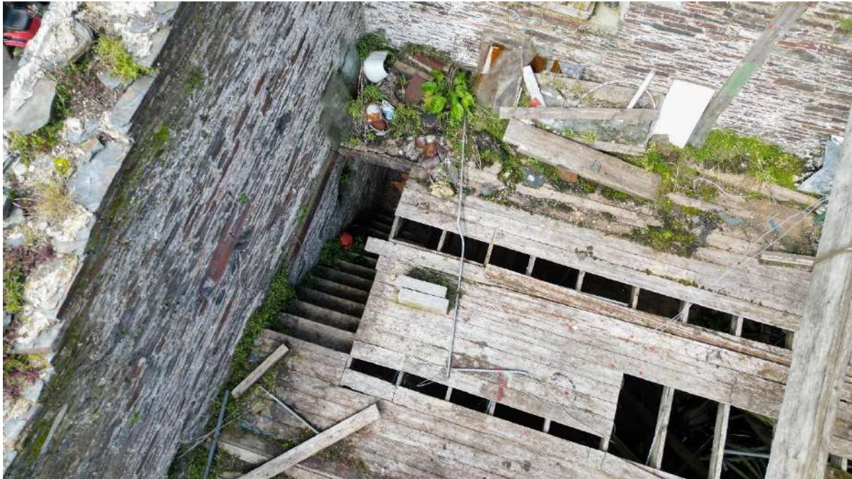
Fig 3.99. Northwest corner with stairs visible
