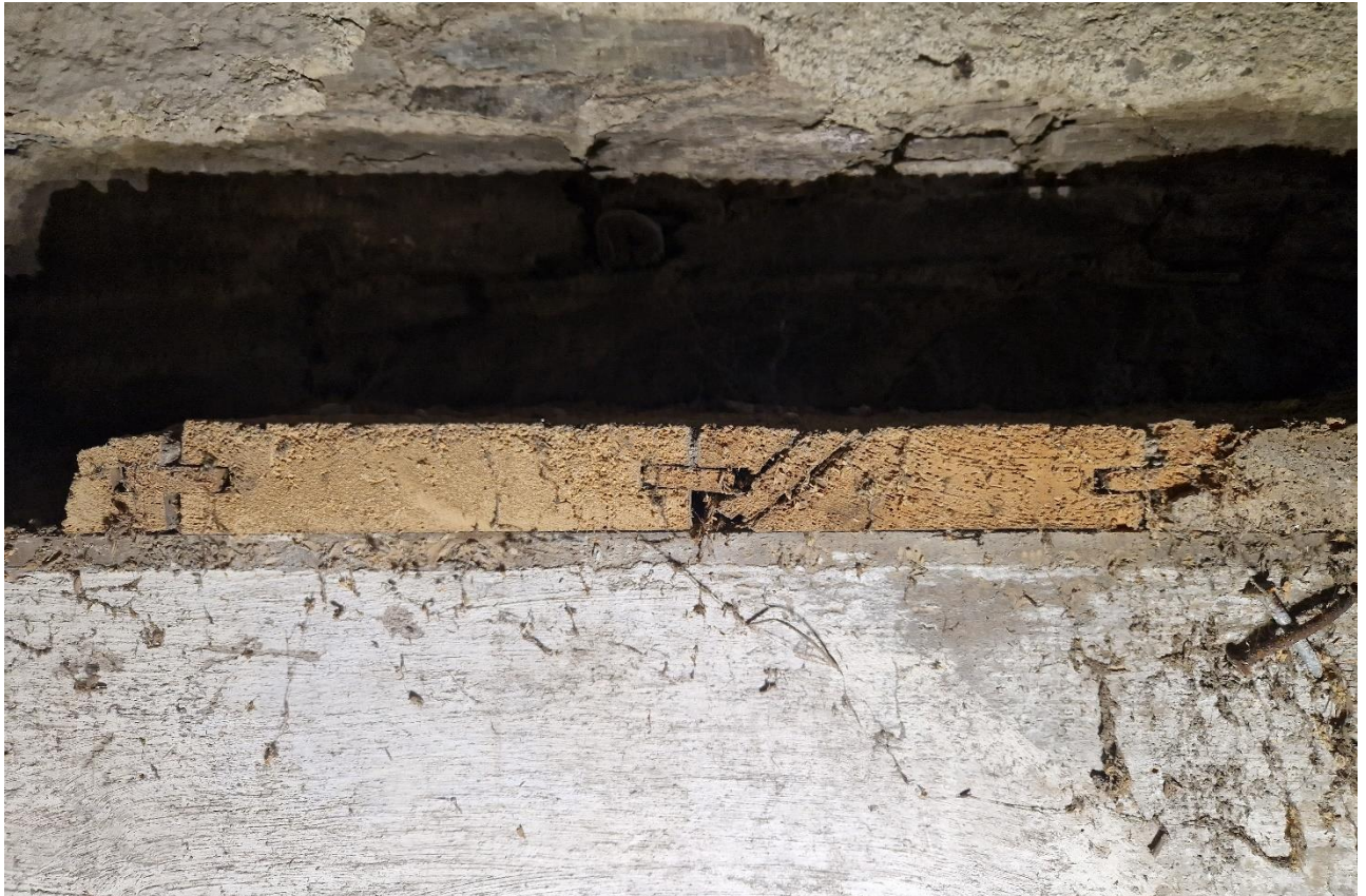
Figure 7. Shows a section through the 'heavy' section floorboards. Note the heavy tunnelling from furniture beetle.
