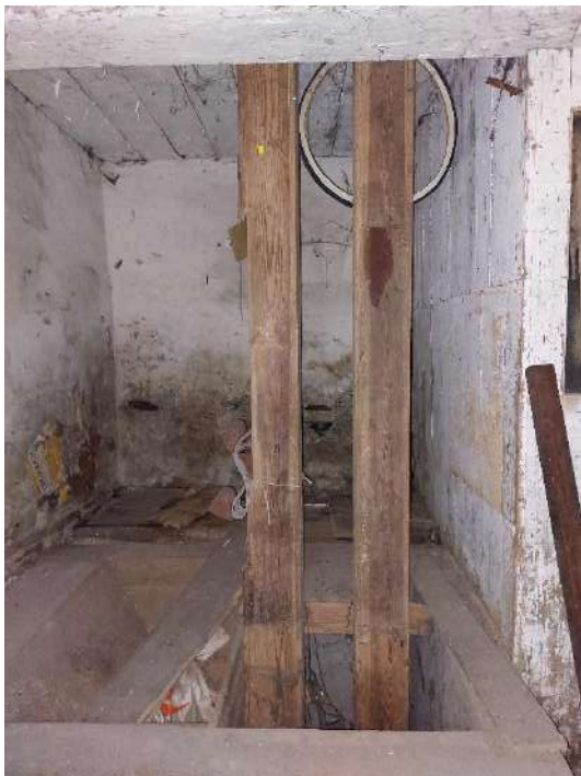
Fig 3.40: Chutes to southwest corner of main volume. Damp to walls behind with mould visible.
