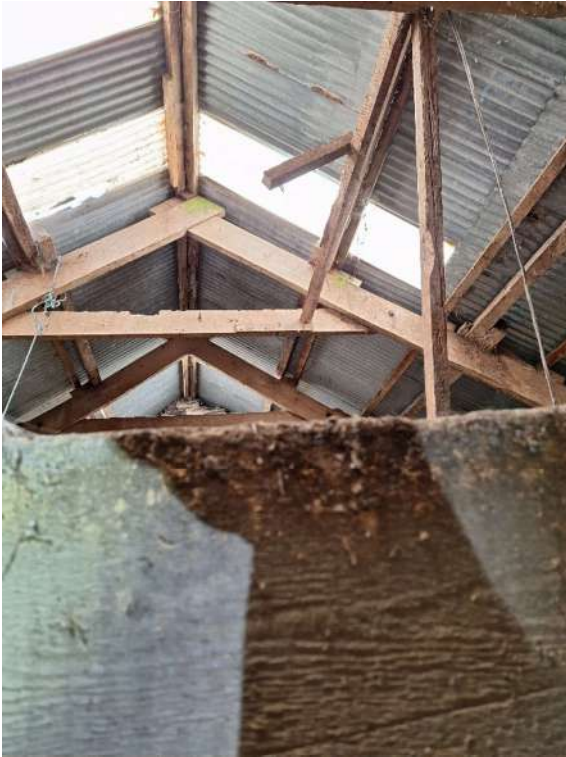
Photo 17 – Corrugated roof and timber truss
