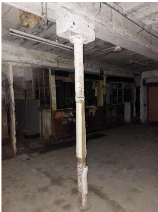
Fig 3.31: Metal post supporting timber structure to west end of building.
