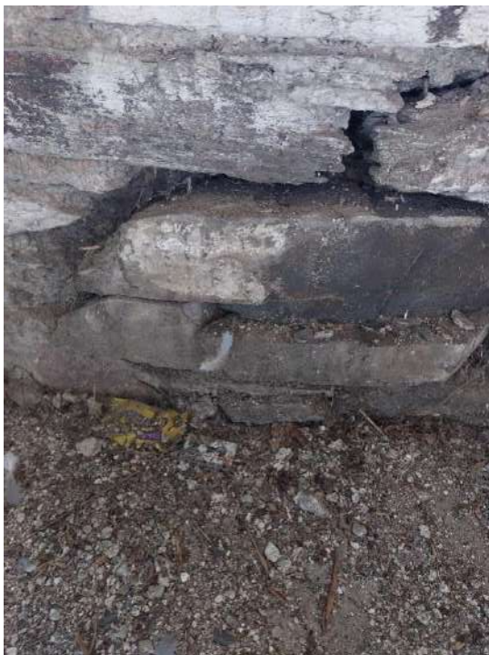
Fig 3.73: Cracking in east wall
