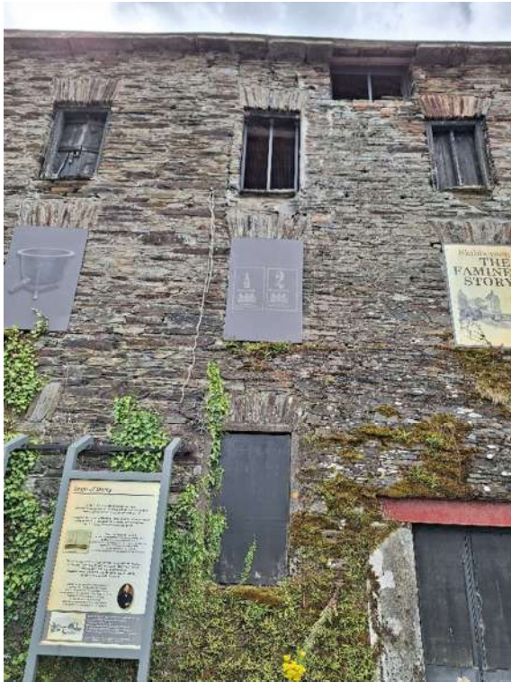
Photo 8 – Northern facing wall showing capping and opt to roof void
