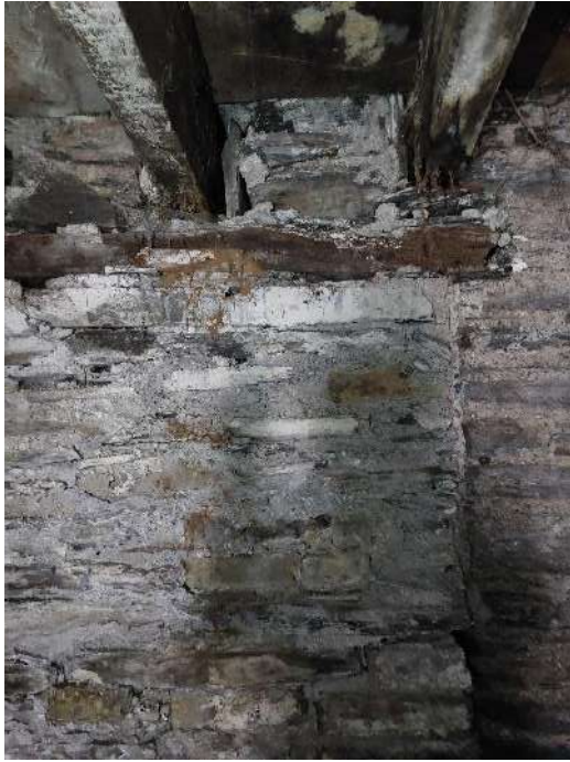
Fig 3.50: embedded joists and lintel decayed to south elevation of west room.
