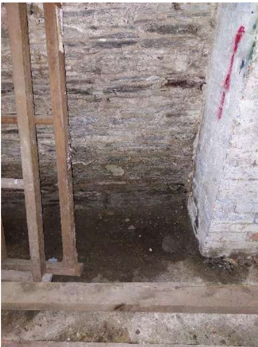
Fig 3.37: Damp visible to ground floor slab and base of external walls
