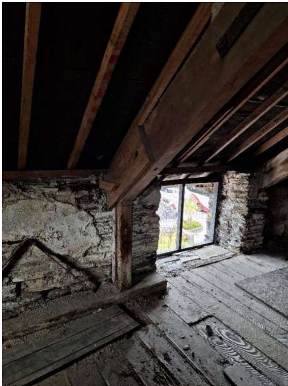
Photo 6 – Second truss base with damp rot showing on original truss
