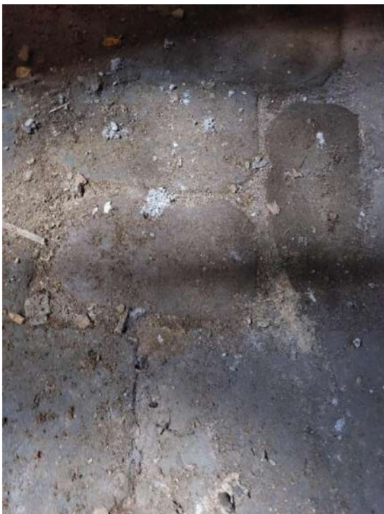
Fig 3.90. Flagstone floor to south annex
