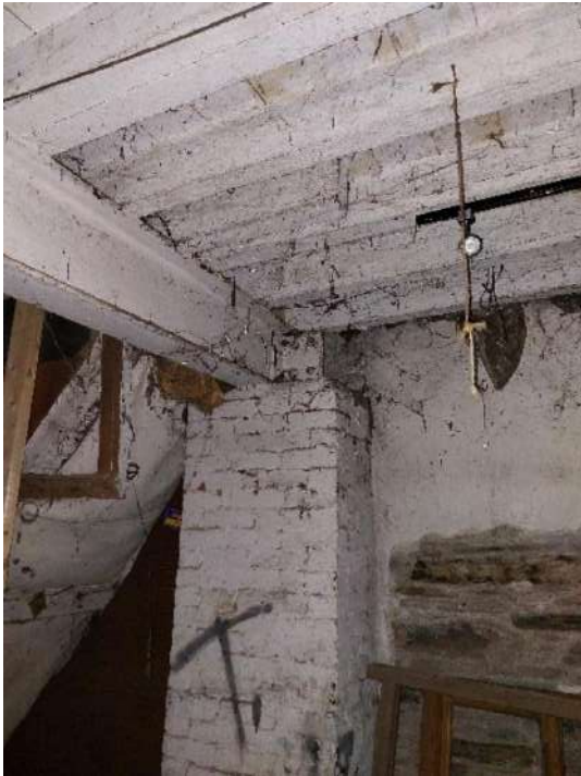
Fig 3.30: Steel structure on brick piers to east end of ground floor
