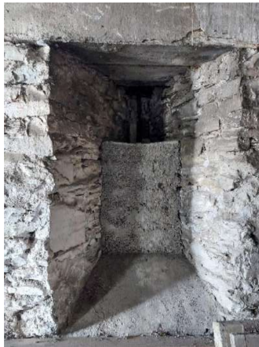
Fig 3.61: Blocked up window opening to south wall.
