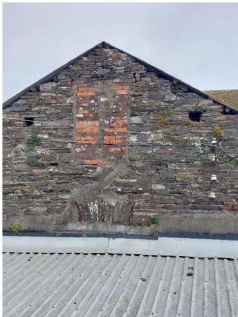
Fig 3.22: South gable wall of south annex
