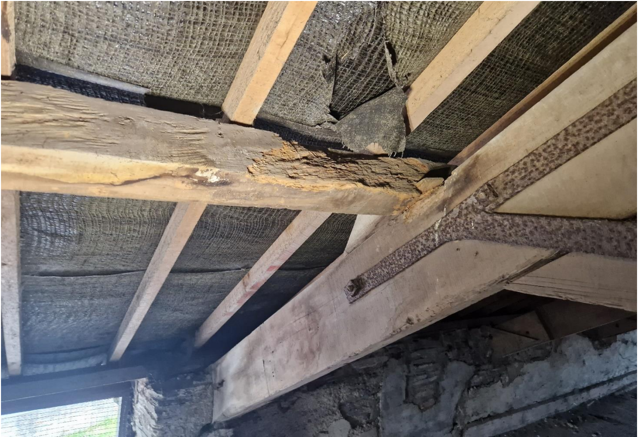
Figure 11. Shows deterioration of a purlin connection.
