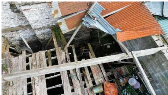
Fig 3.100. South east corner with remains of corrugated roof structure
