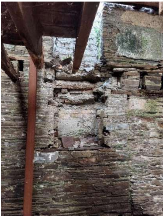
Fig 3.97: Opening / infill section in west wall with steel post visible
