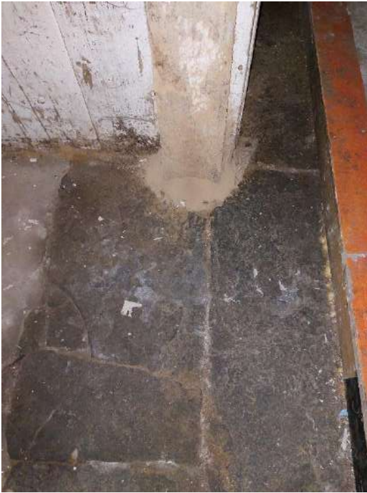
Fig 3.35: Flagstone to west and of main volume ground floor
