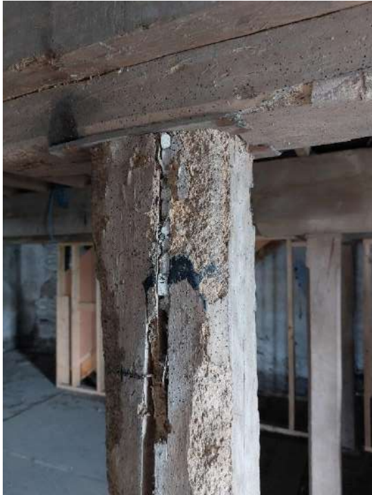
Fig 3.69: Timber beam and column with woodworm damage visible
