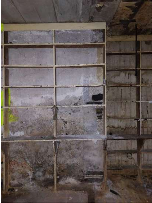
Fig 3.39: West wall of shop with fitted shelving
