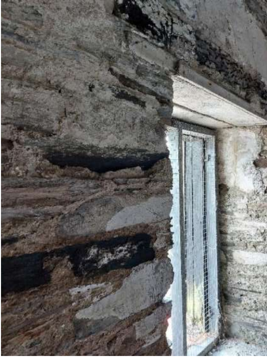
Fig 3.82: View of east wall window opening
