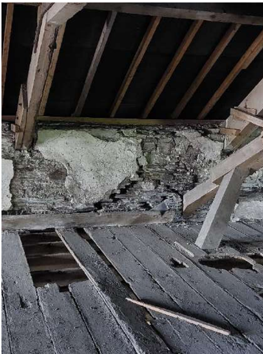
Fig 3.76: View of third floor facing south
