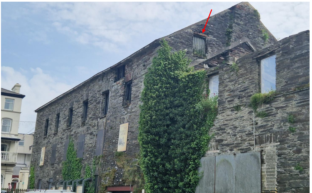
Figure 6. It highlights the poor condition of the exposed lintel on the north of the west gable that should be replaced.
