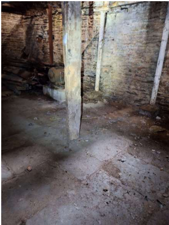
Photo 20 – Example of condition of timbers
