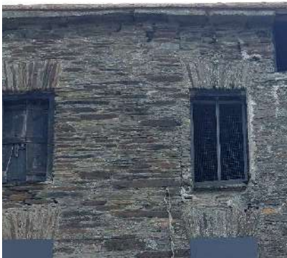
Fig 3.11 Detail of stonework- eroded joints and cracking visible, especially at eaves level
