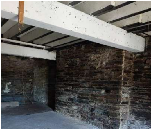
Fig 3.33: View of chimney breast to west room with timber structure above.
