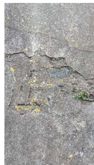
Fig 3.09: Failure of render finish
